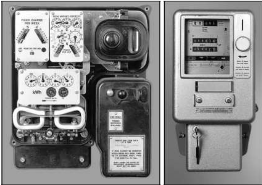
Fig. 1–24. An obsolete coin meter. (Photo by Landis+Gyr.)
