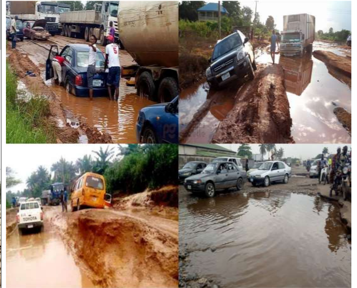
Bad Constructed Road in Anambra State, 2021
